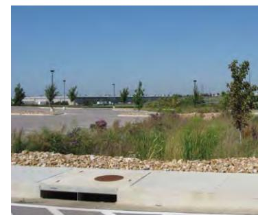
Street drainage flows into this roadside bioswale in Lenexa, Kansas. The city found that on-site detention with LID practices cost 25 percent less than traditional stormwater management retrofits.
